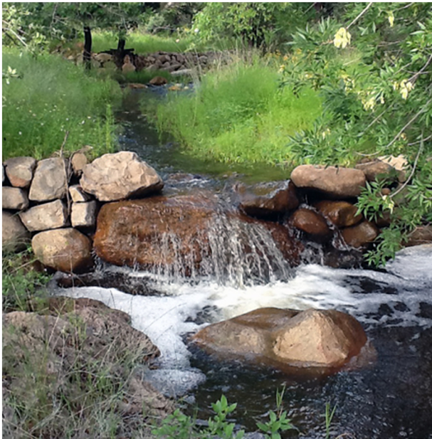
Figure 1. Photograph of check dams in the Turkey Pen sub-watershed of West Turkey Creek, southeast Arizona. This figure is available in colour online at wileyonlinelibrary.com/journal/rra
